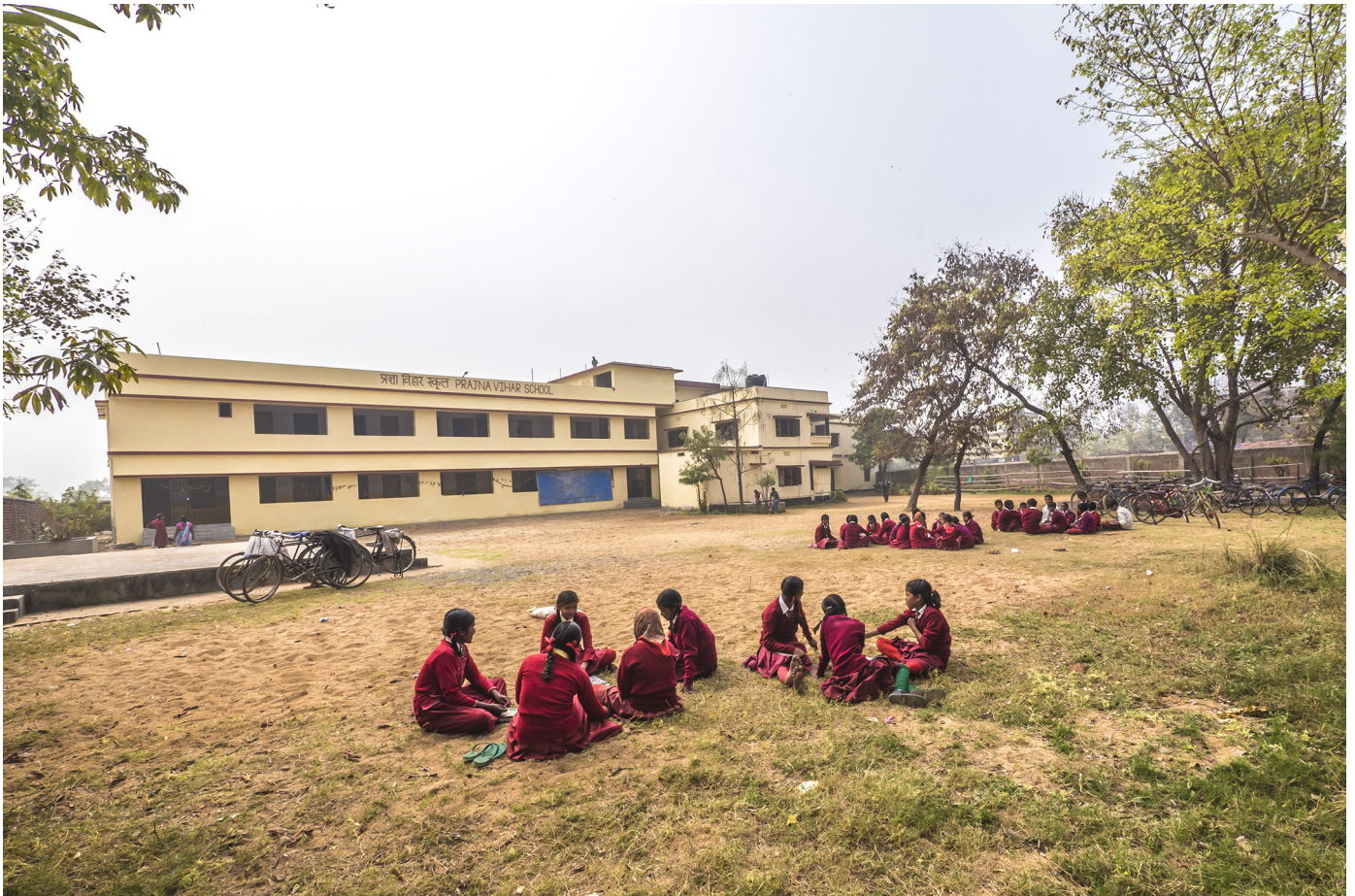
Our newly constructed wing is on the left
